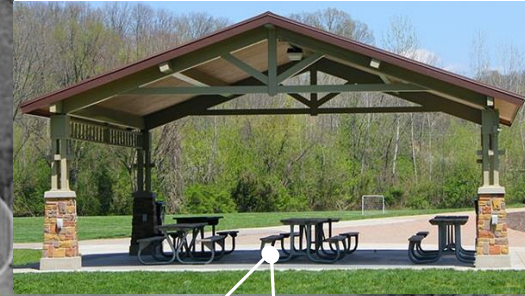
NEW LARGE SHELTERS
